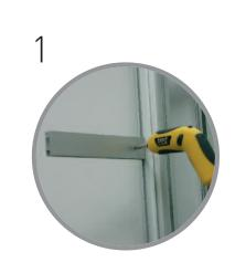
Locate 220mm straight profile in desired position and insert into 8-way post. Secure by tightening expanding clamp grub screw.
